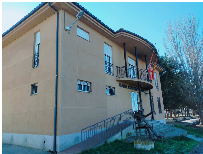
Fachada principal – norte
